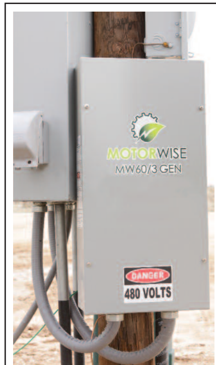
The MOTORWISE™ controller from the TechnoWise Group is designed to reduce electricity costs by monitoring pumpjack loading and automatically adjust the amount of electricity supplied to the motor based on specific load requirements at any given point in the cycle.
